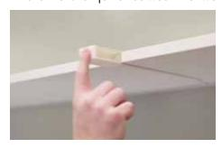
• In the case of abutting two shelves at right angles in the corners, insert the second shelf into the backwall channel before sliding the corner H-channel shelf joiner between the two shelves.
