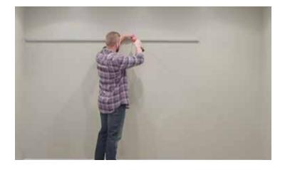
B Install Sidewall Bracket and Universal Pole Cup
